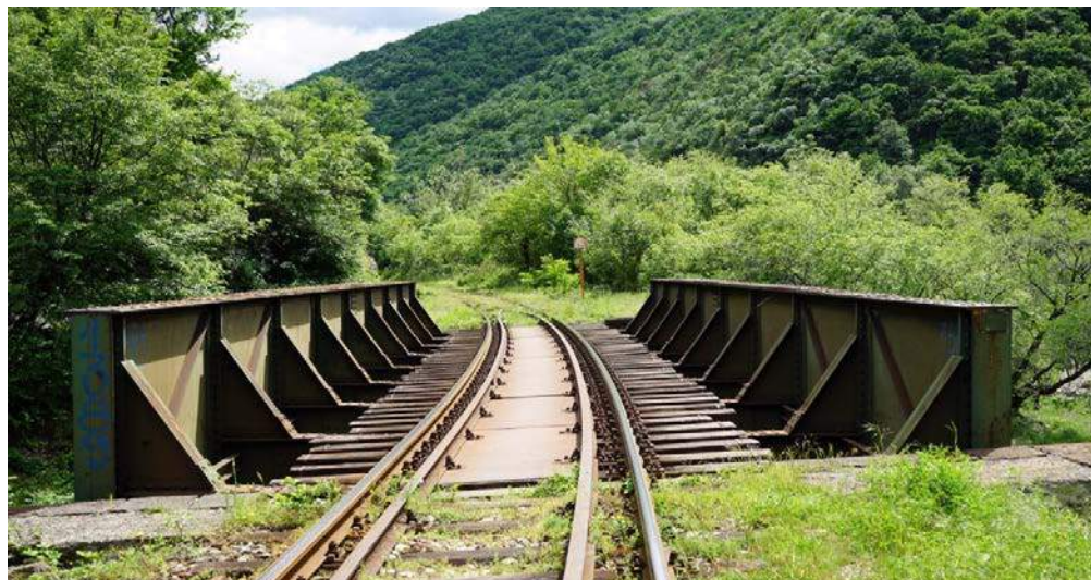
View of Non-electrified Railway Track on Corridor Xc, Serbia.
