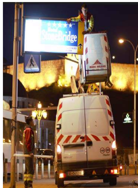
Installing LED lighting in Skopje, the former Yugoslav Republic of Macedonia.
