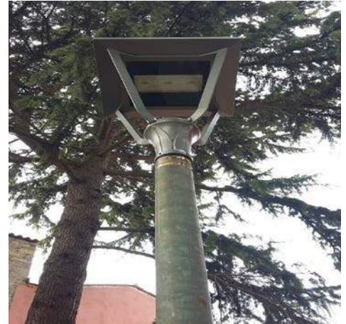
Mounting of New LED Lanterns in the Old Town of Novigrad, Croatia
